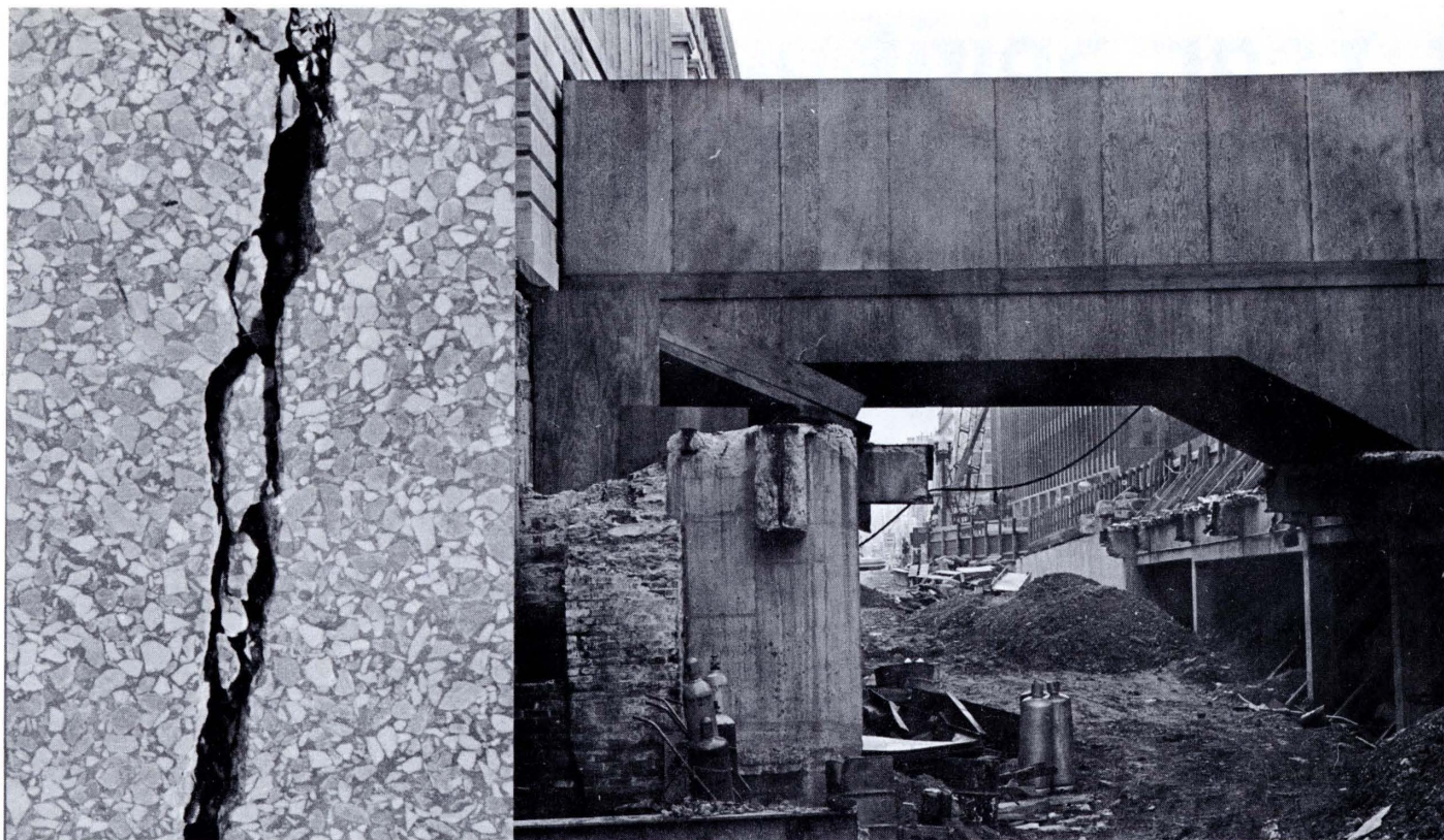
Inside the NCFA, a crack crosses the Lincoln Gallery terrazzo floor; outside, work proceeds on the 55-foot deep subway trench. Photographs by John Bergner
