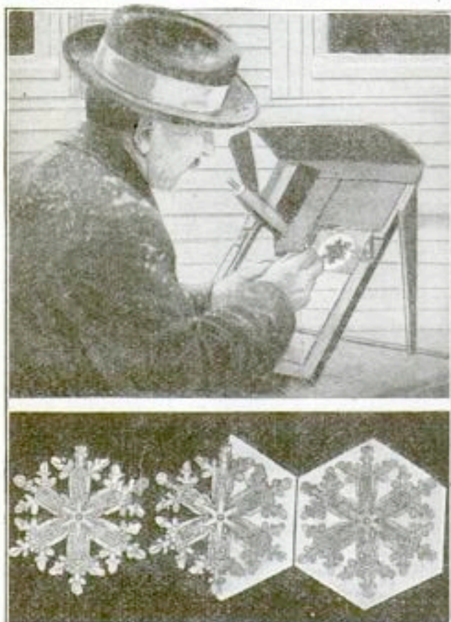
Blocking Out the Snow-Crystal Images on the Photographic Negative: Right, Original Negative; Center, Negative Partly Blocked Out; Left, Completely Blocked-Out Negative
