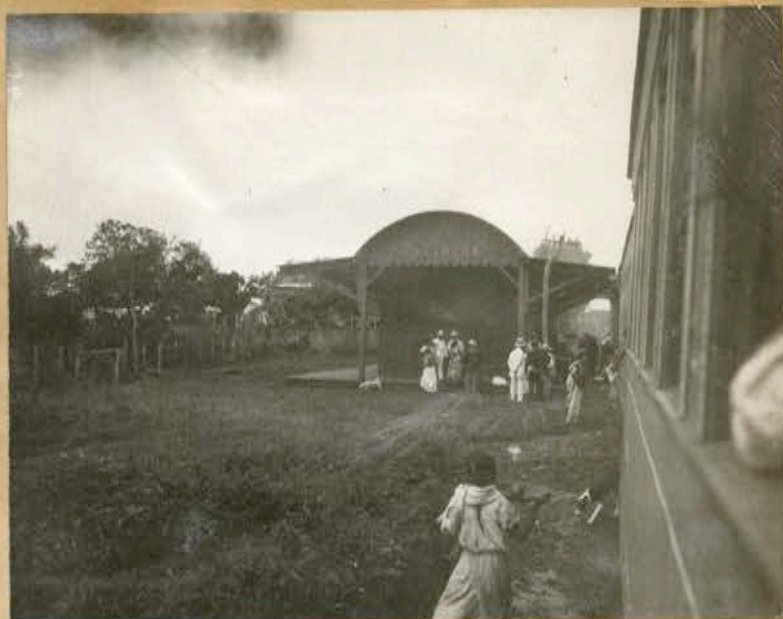
179 Railway Station Catarinas
