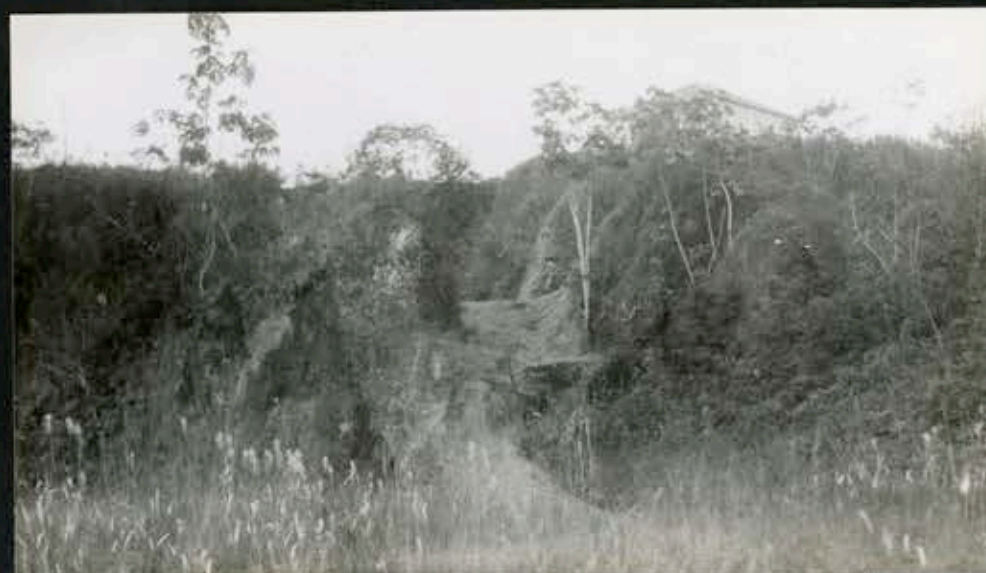
1868. Lavras, showing erosion in red clay hills.
