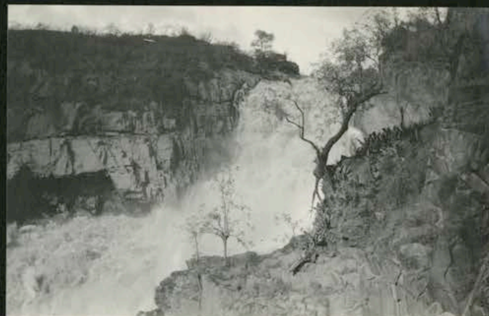
1801. Paulo Affonso falls from turbine station.
