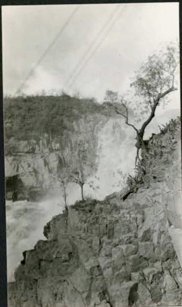
1799. Paulo Affonso falls from turbine station.
