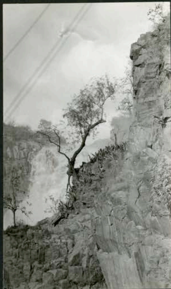
1800. Paulo Affonso falls from turbine station.
