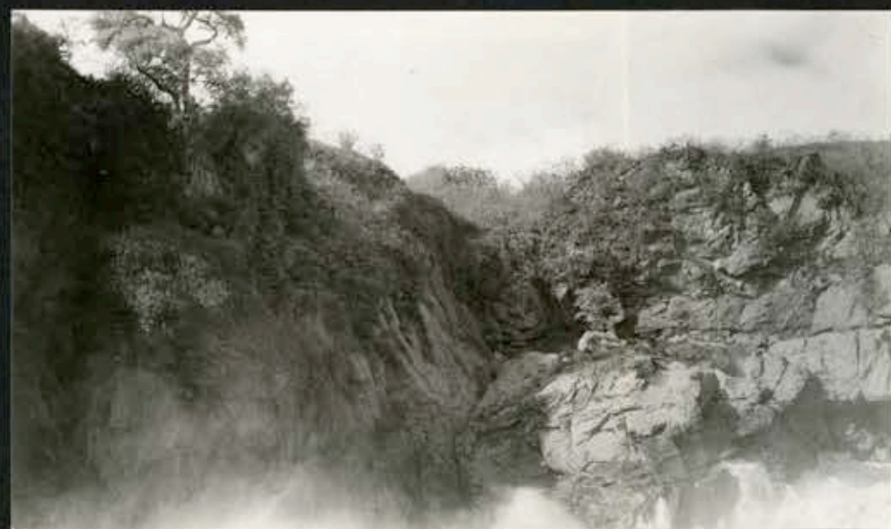
1803. Paulo Affonso falls from turbine station.
