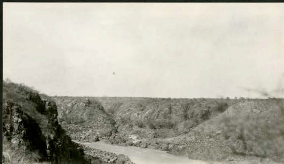
1827. Stream separating power station from mainland.
