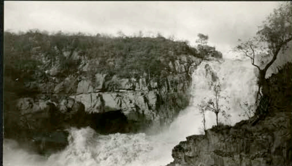
1794. Paulo Affonso falls from turbine station.
