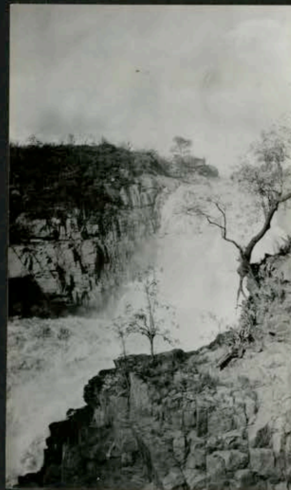
1802. Paulo Affonso falls from turbine station.
