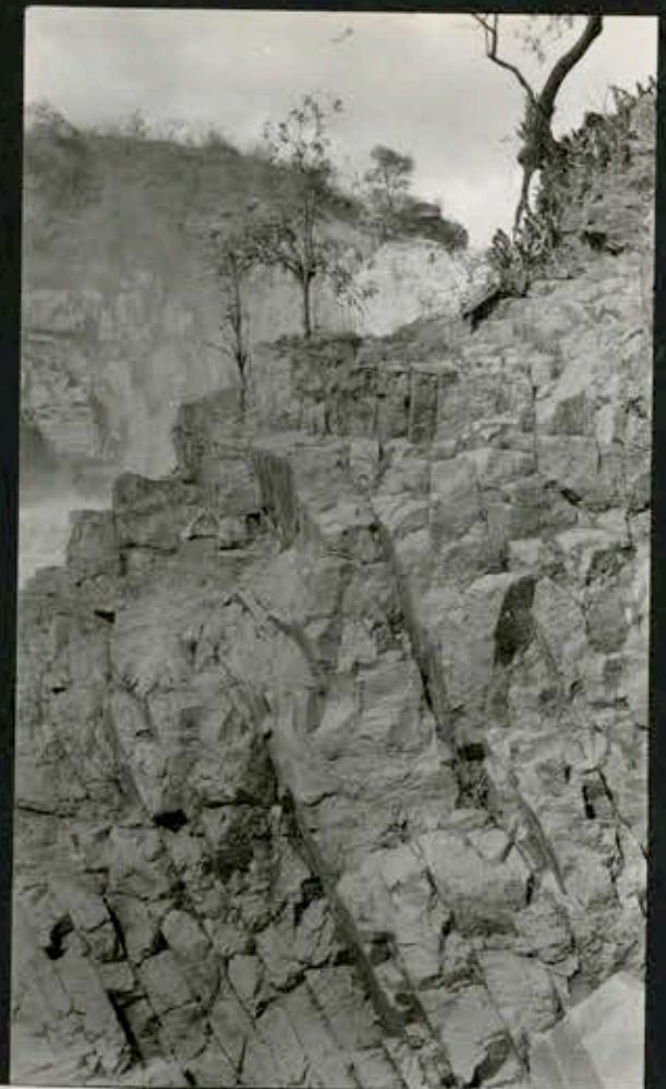
1805. Paulo Affonso falls from turbine station.
