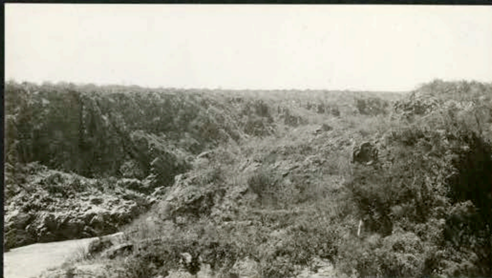
1820 2 . Stream separating power station from mainland.
